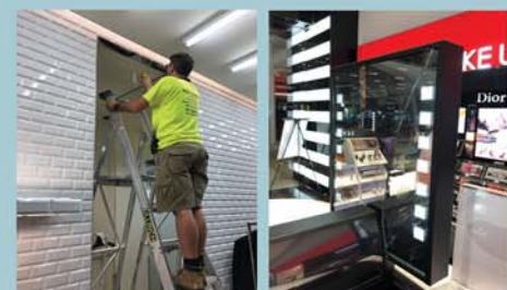
Paint touchups and repairing broken glass
