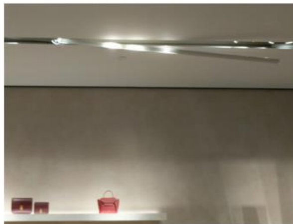
E.G. Emergency shop fitting and electrical repairs
