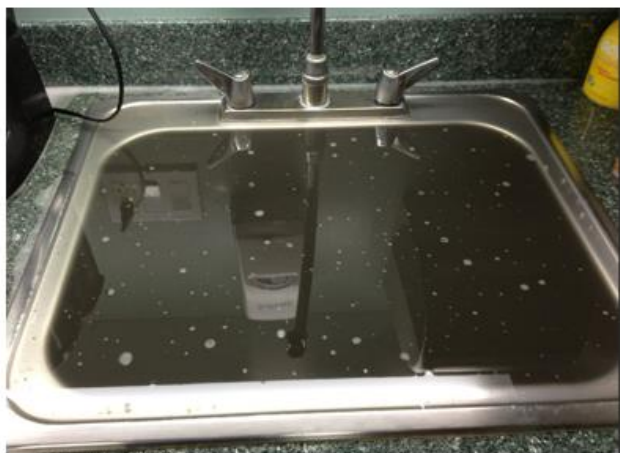
E.G. Emergency plumbing issues solved
