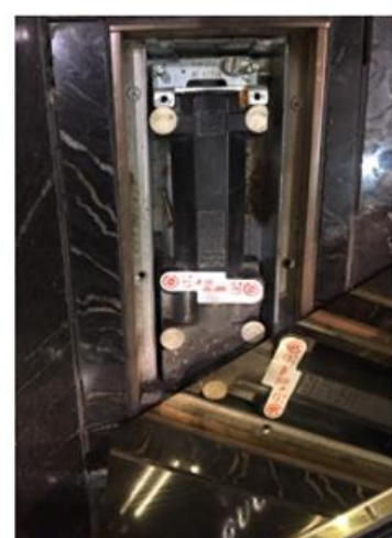
Lock and hinge check, clean, lubricate
