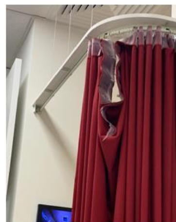
Curtain and track repairs/replacement
