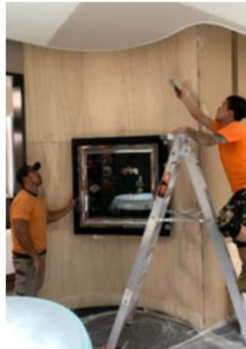
Manufacture and installation of specialized millwork
