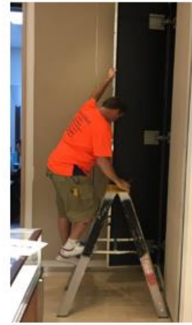
Replace mirrors and repair cabinetry
