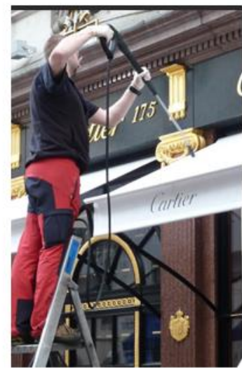
Awning pressure cleaning
