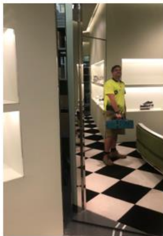
Repair floor tiles and other floor coverings
