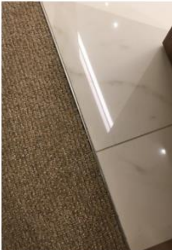
Supply and installation of new floor coverings
