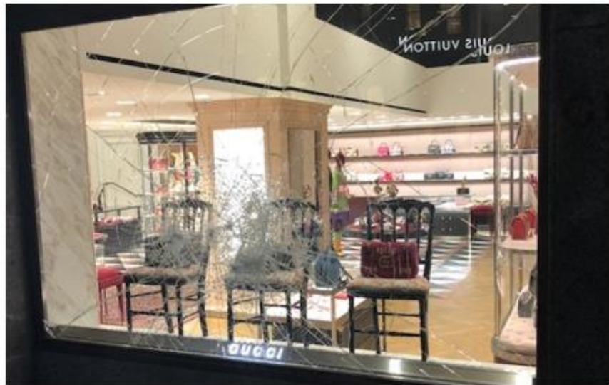
E.G. Emergency glass repair - we will arrange security and glass replacement
