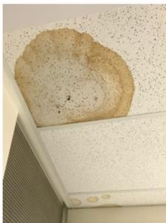
Ceiling tile replacement
