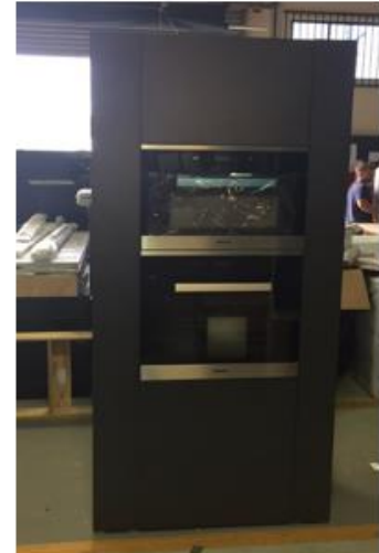
Manufacture and installation of cabinetry
