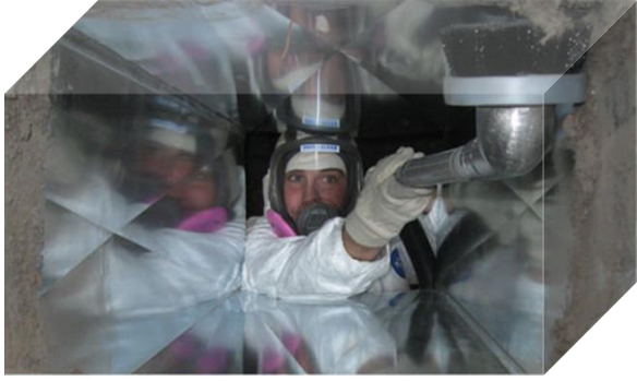
AC duct deep cleaning
