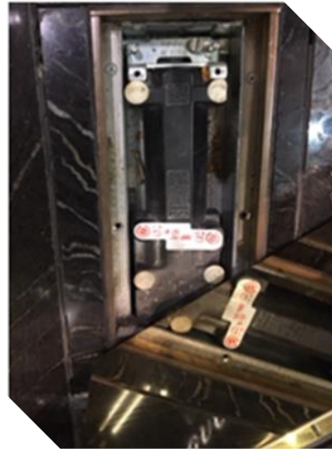
Lock & hinge check, clean, lubricate
